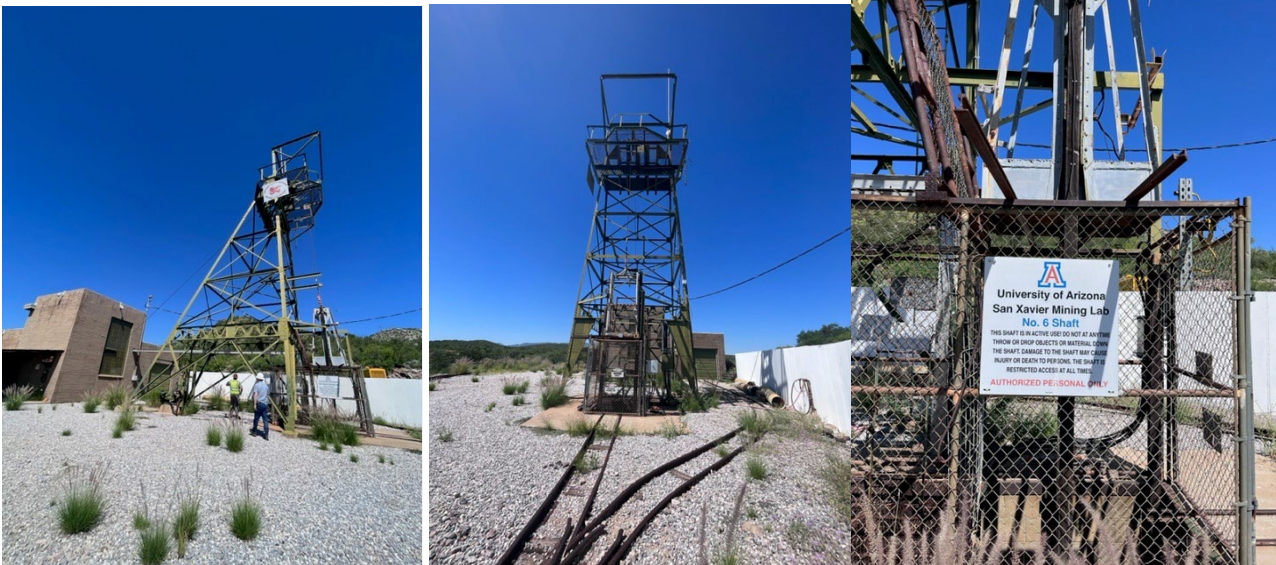
No.6 Shaft and Hoist headframe views
