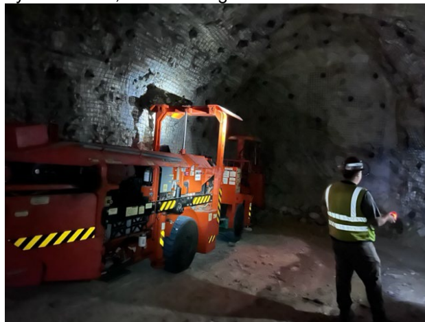
Drill on working face
